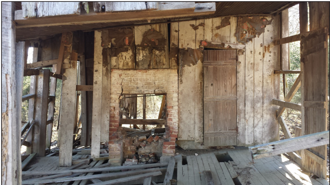
Figure 3. Room I of SCH#1, facing south.
