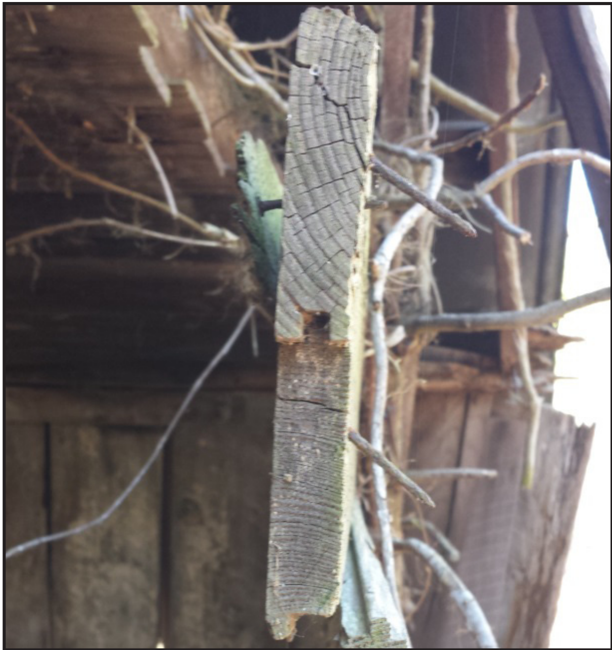
Figure 27. Tongue and groove boards used in the construction of interior walls of a structure.
