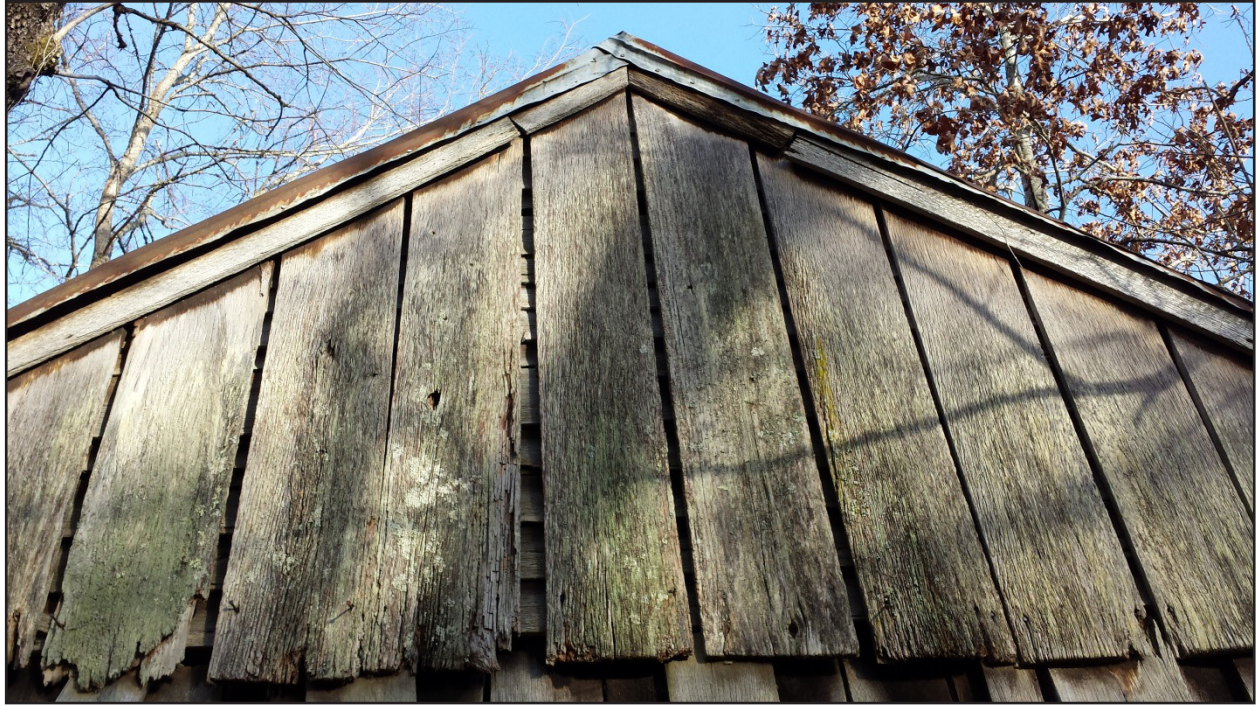
Figure 30. Clapboard siding underneath the board and batten on the gable of SCH#6.
