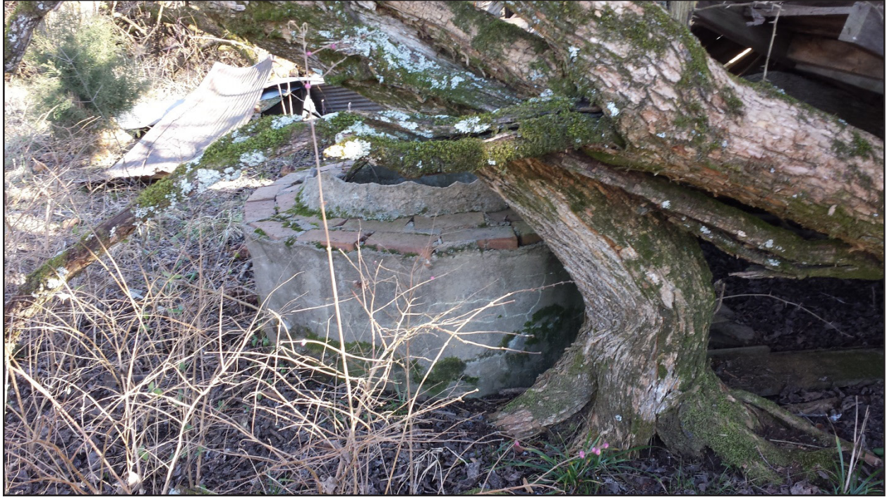
Figure 6. General view of the cistern located on the northwestern side of the SCH#2.
