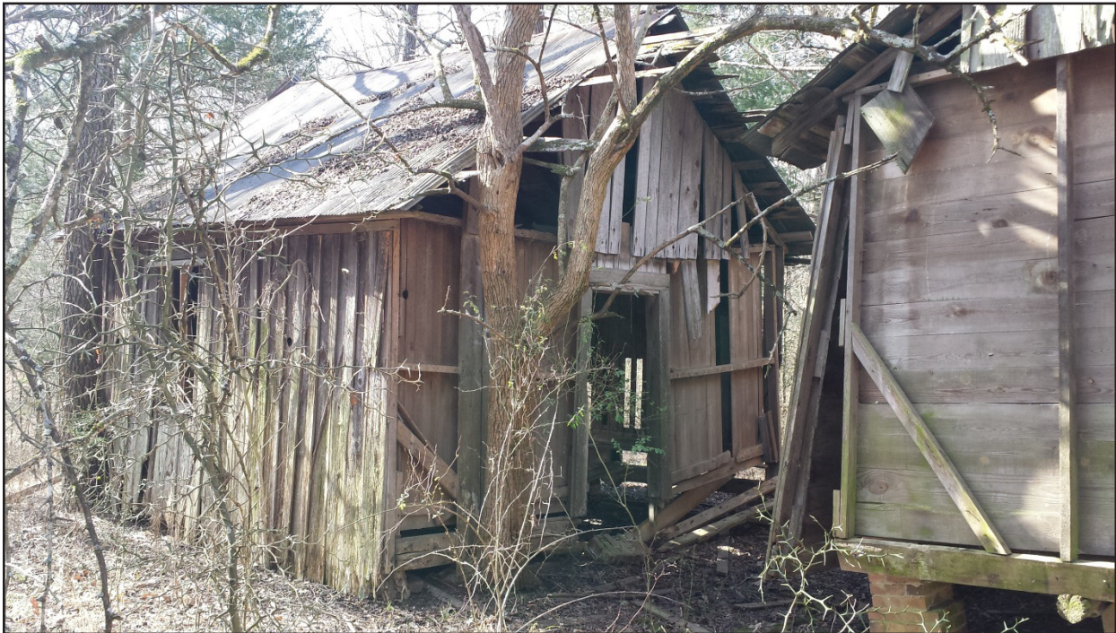
Figure 15. View of the detached kitchen for SCH#5.
