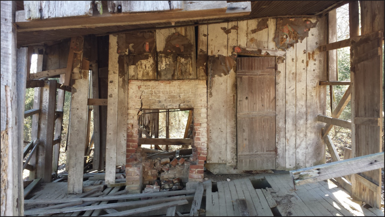
Figure 24. Central chimney with a double fireplace.
