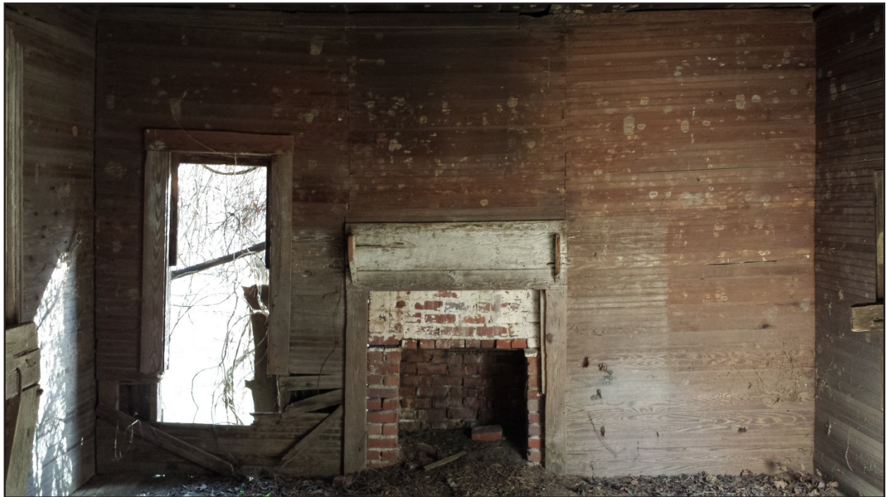
Figure 12. The east wall of Room II in SCH#4.
