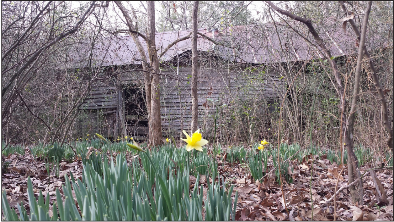
Figure 32. General view of SCH#11.
