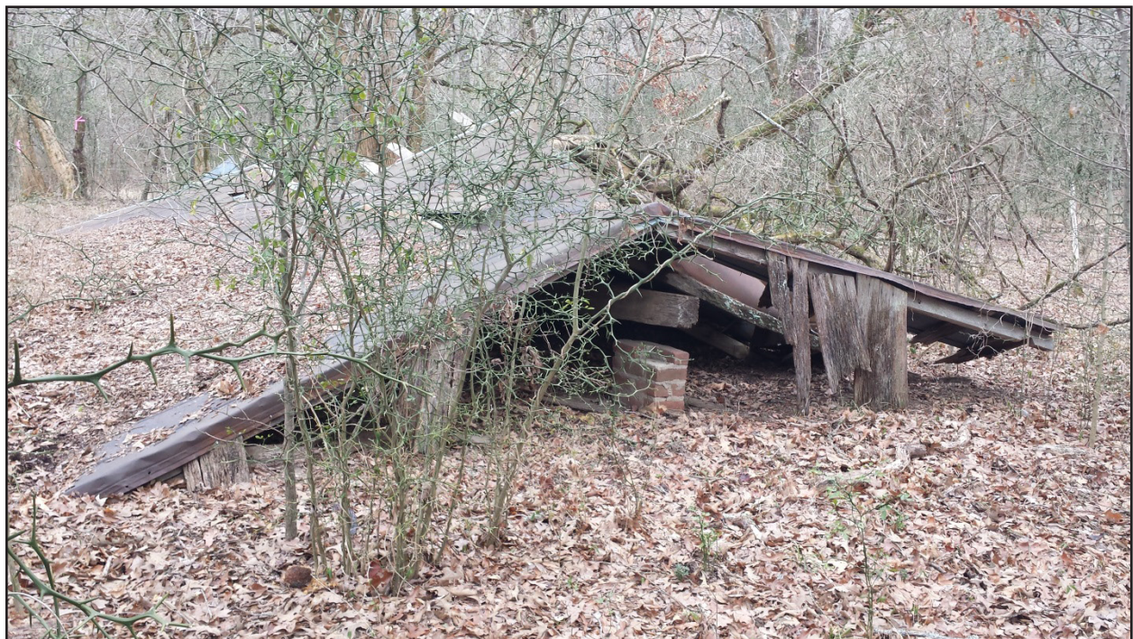
Figure 29. General view of SCH#10.
