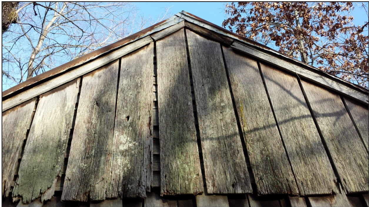
Figure 18. View of clapboard underneath the board and batten on the backside of the gable on SCH#6.
