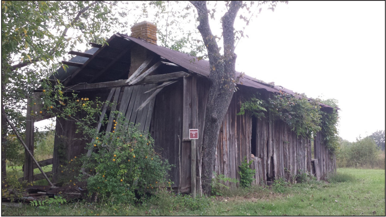
Figure 8. General view of SCH#4.
