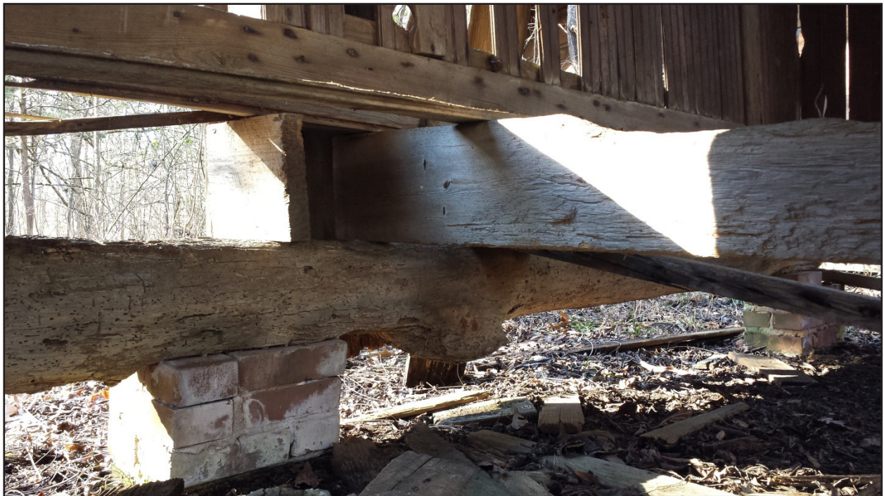
Figure 17. Types of sills used to hold up frame of structure (milled wood beams and an unmodified tree).
