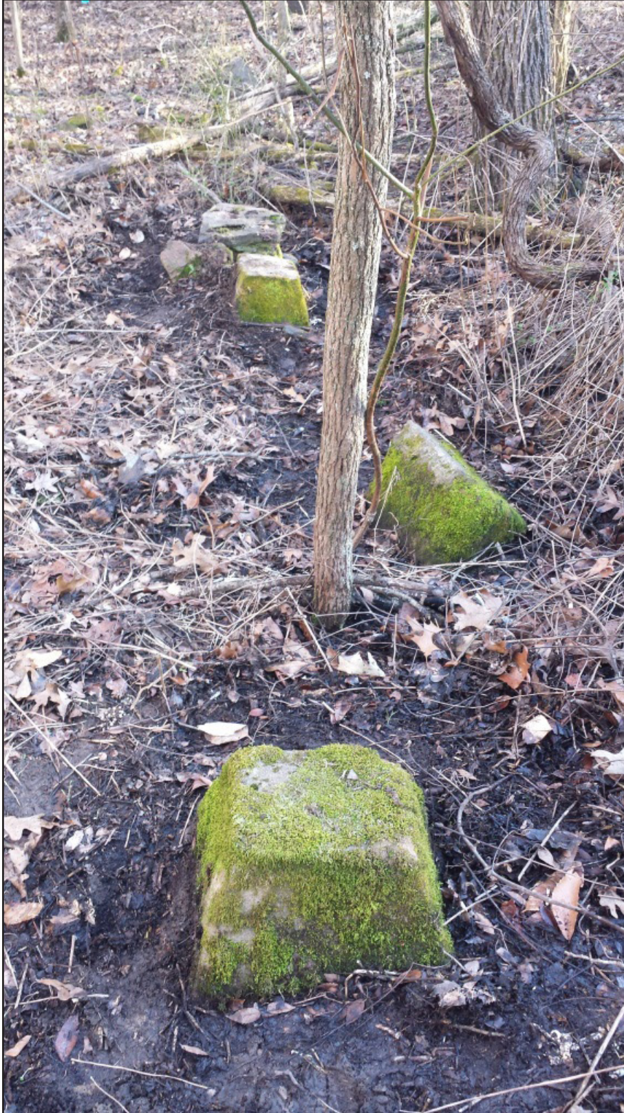
Figure 48. Concrete blocks and sandstone used as foundations for SCH#16.
