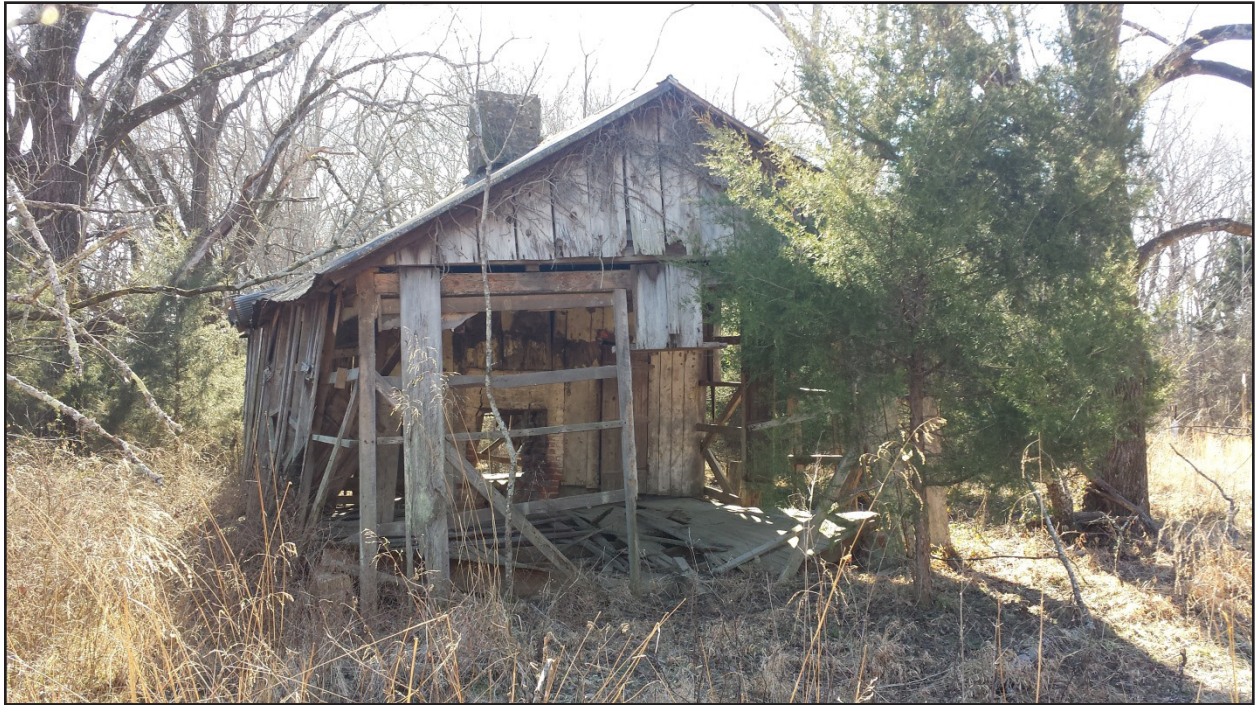
Figure 2. General view of SCH#1, facing south.
