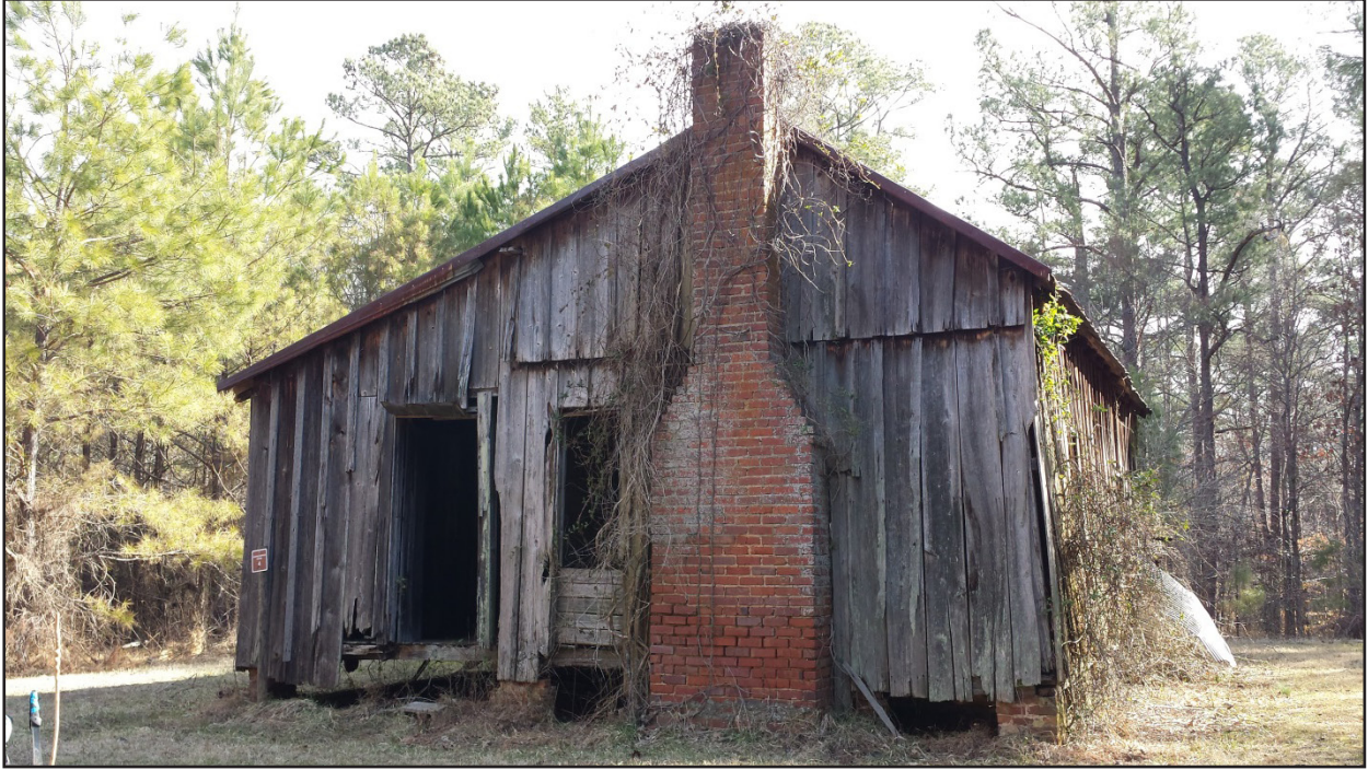
Figure 23. End gable chimney with a single fireplace.
