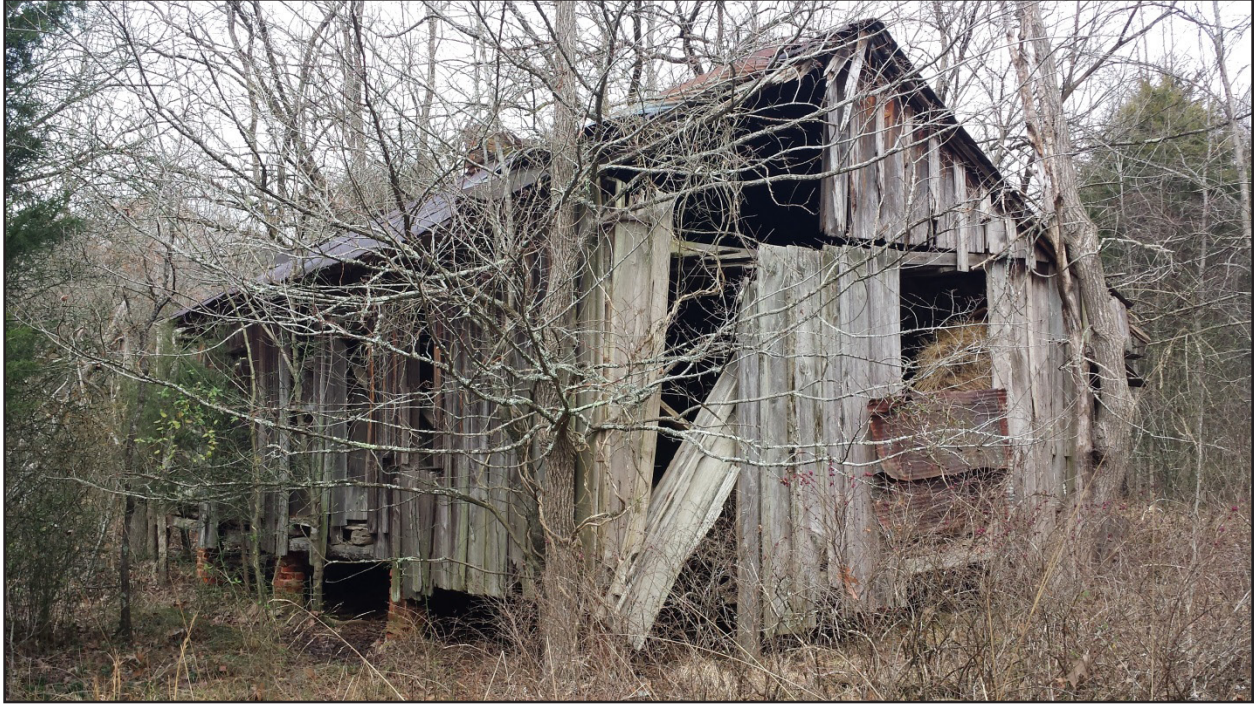
Figure 26. General view of SCH#9
