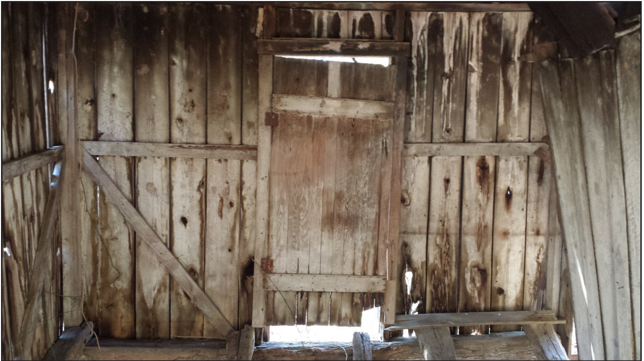
Figure 21. The west wall of Room III in SCH#7.
