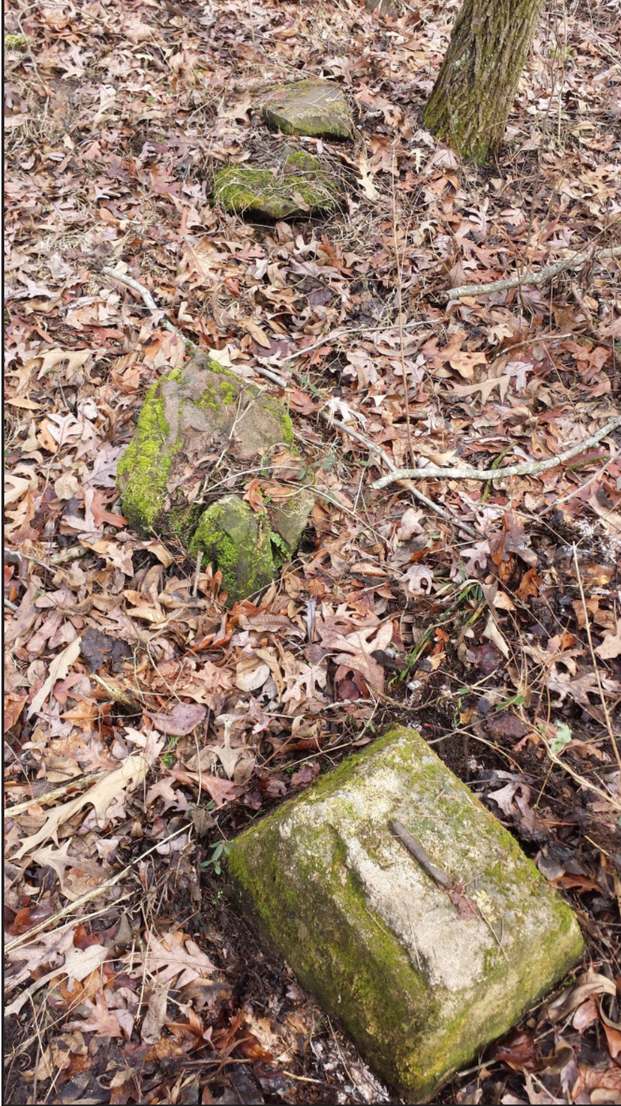
Figure 42. Concrete block and sandstone used as a foundation for SCH#14.
