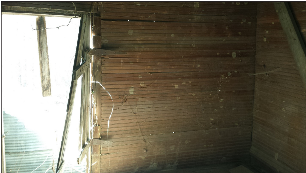
Figure 26. Bead board on the interior walls of a structure.
