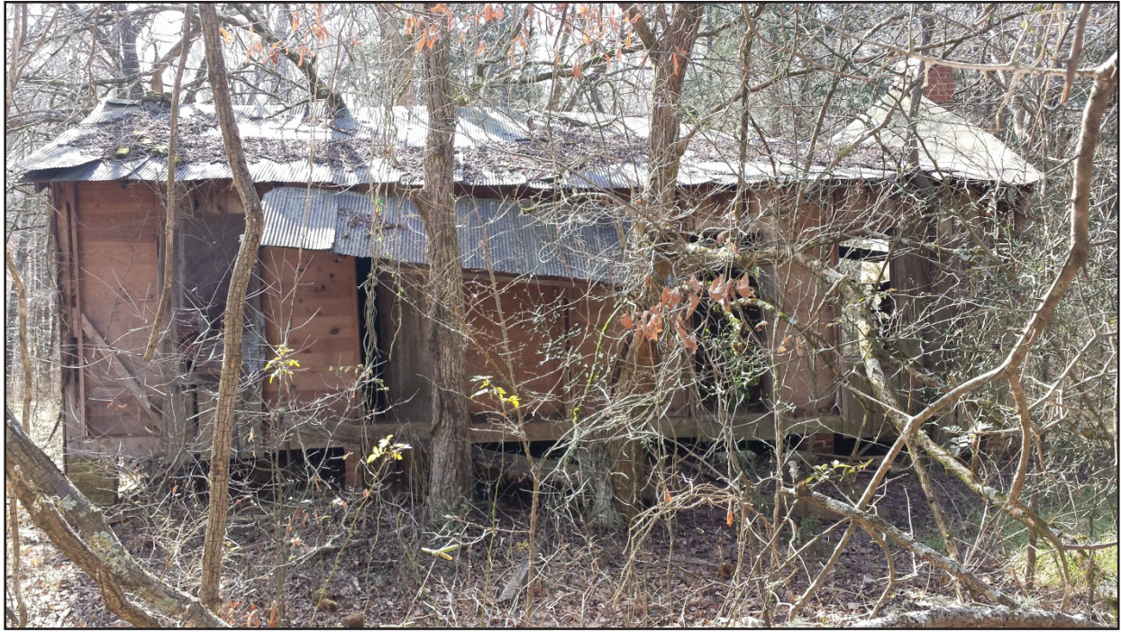
Figure 14. General view of SCH#5, facing south.
