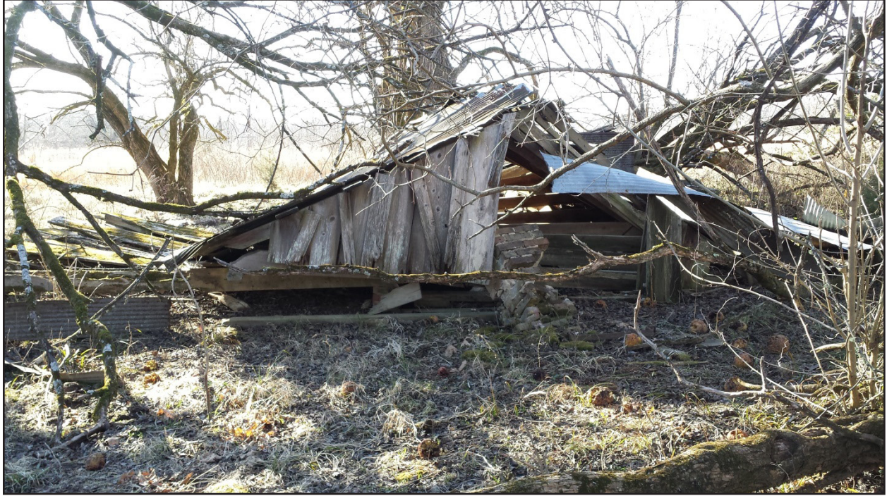
Figure 5. General view of the east side of SCH #2, facing west.
