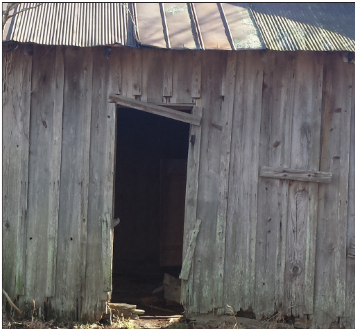
Figure 18. Board and batten siding.
