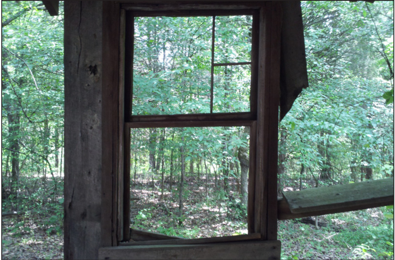
Figure 21. Single hung sash window in SCH #7.
