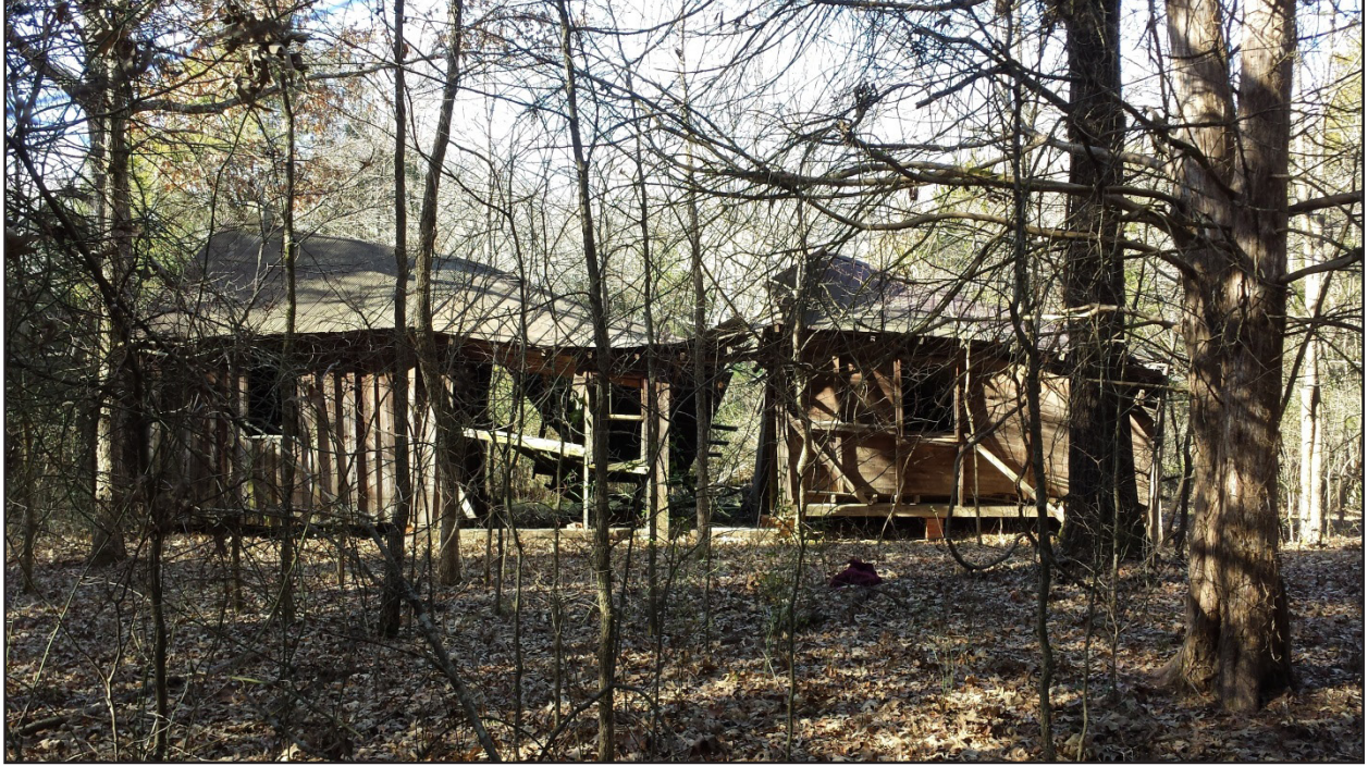
Figure 20. General view of SCH#7.
