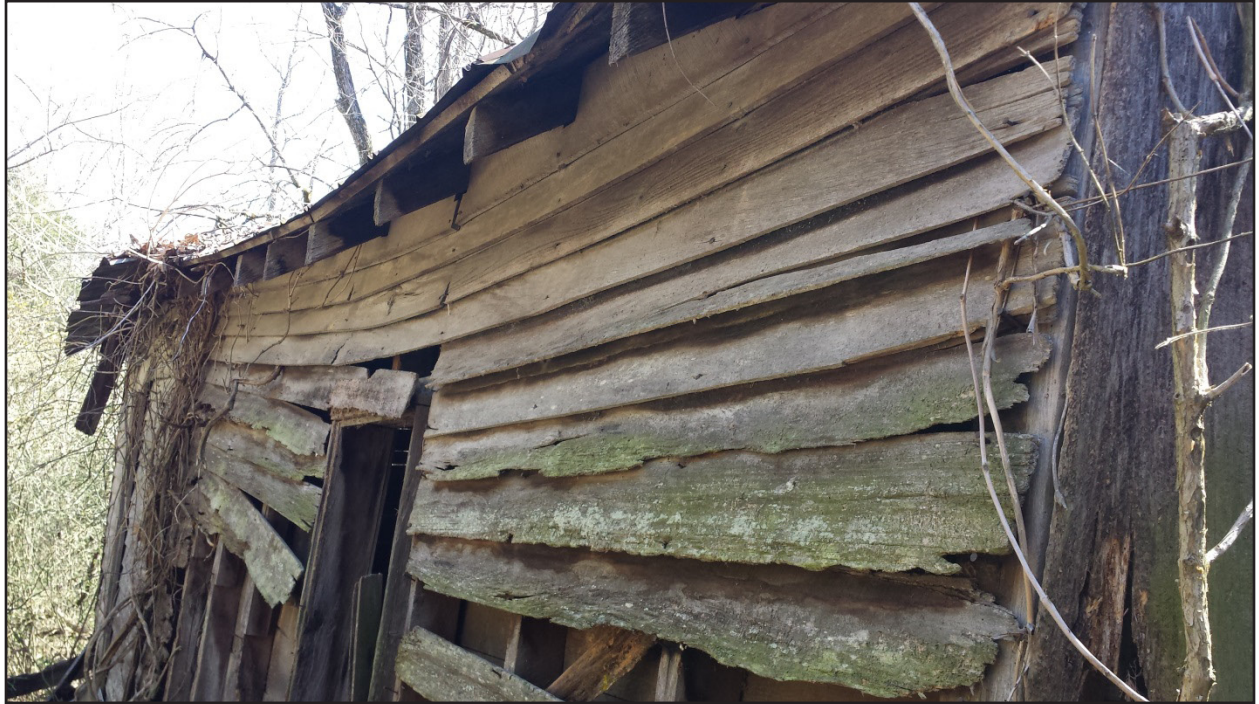
Figure 19. Clapboard siding.
