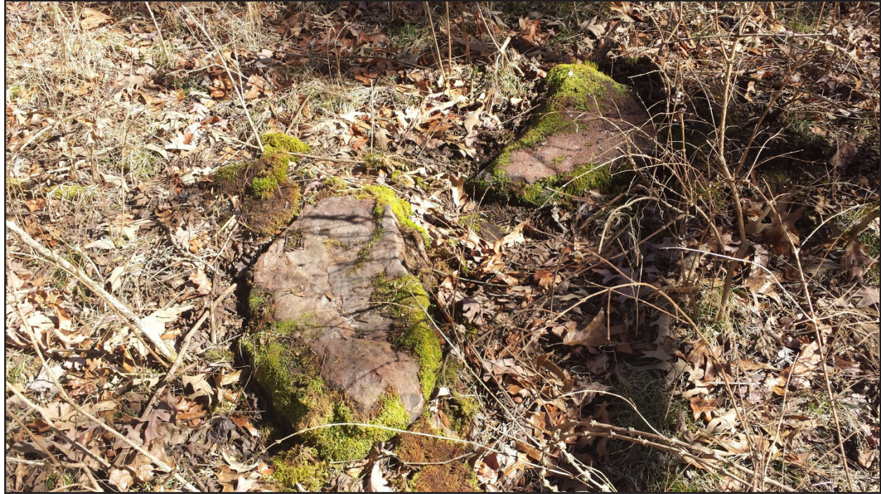
Figure 45. Sandstone foundations found at the area for SCH#15.
