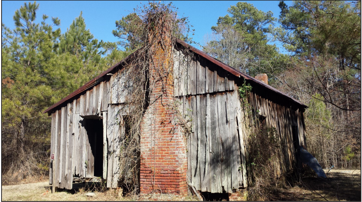
Figure 11. General view of the west side of SCH#4.
