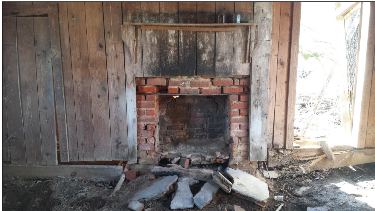
Figure 9. The south wall of Room II in SCH#3.
