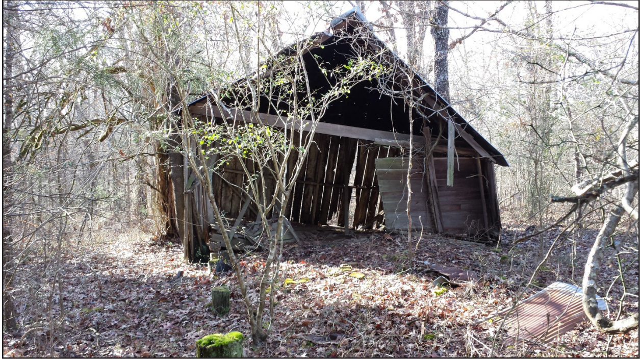
Figure 17. General view of SCH#6.
