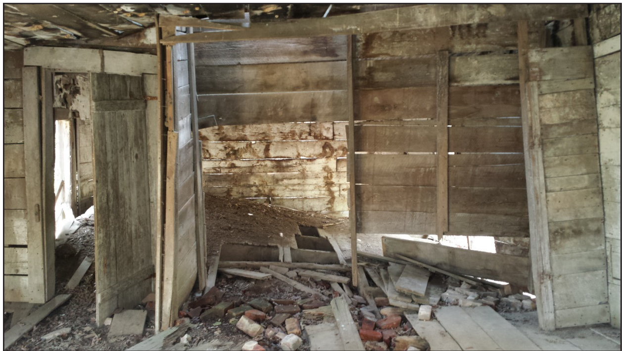
Figure 33. View of Room II from Room I in SCH#11.
